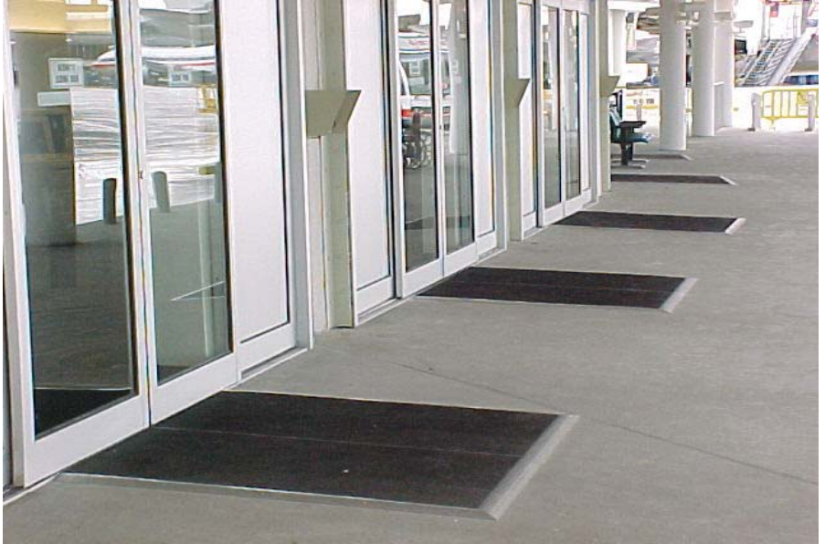
The Miami International Airport uses Larco mats to activate automatic doors allowing customers safe and easy access to their facility.
